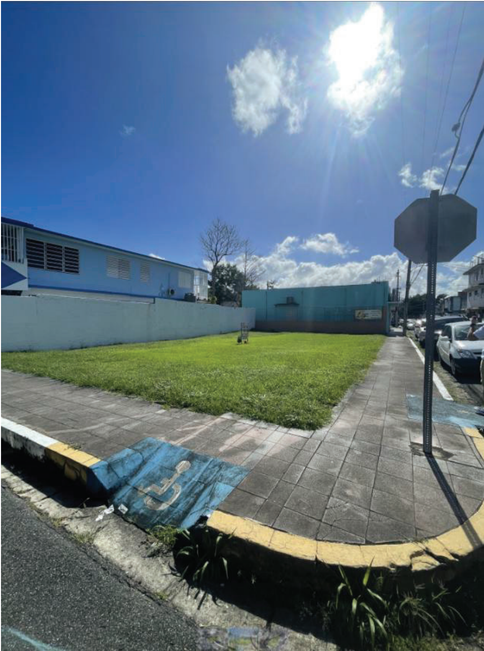
Figure 11. Site conditions, general view. (Source: Hernández-Bauzá PSC Architects, 2025).
