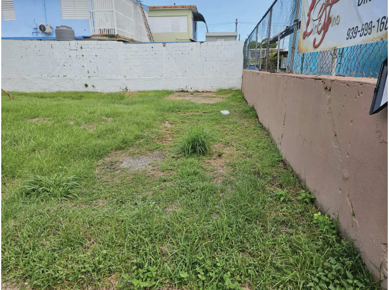
Photograph 3 – Subject/Target property southern boundary. Looking west to east.
