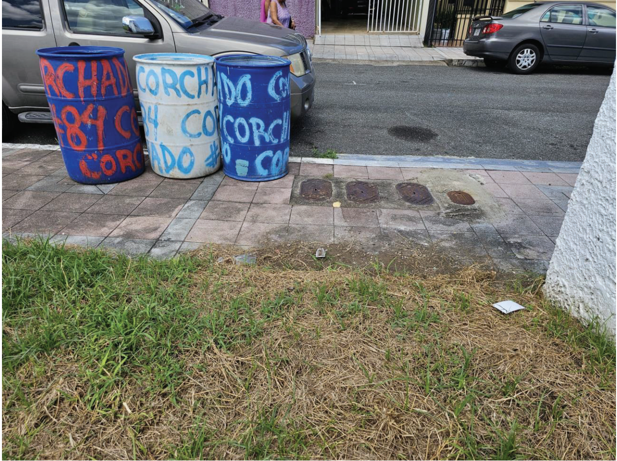
Photograph 8 – Water meters located northeast of the property.
